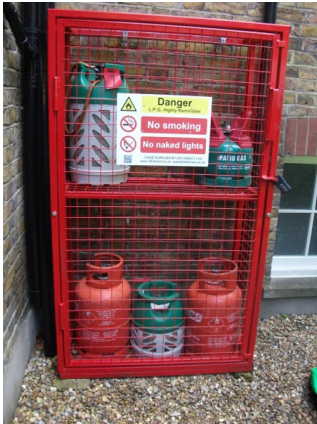
Designated cylinder cabinet outside block 13.
