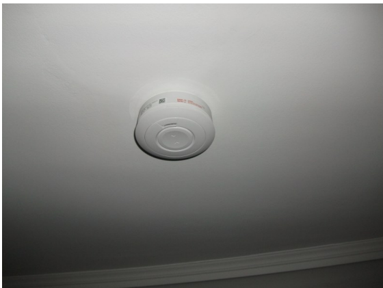
Detection in escape stairways.
