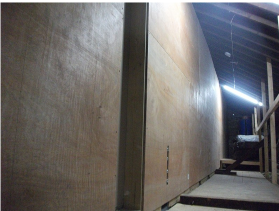
Roof space under development in block 10.
