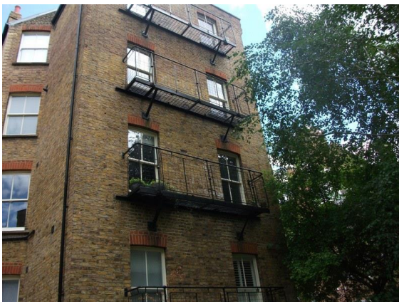
Balconies to rear of building.
