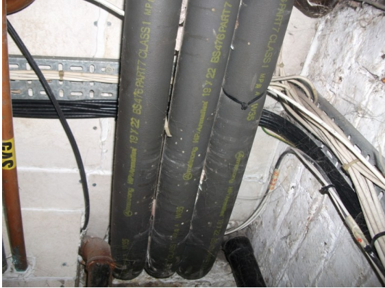
Example of fire separation in basement corridor.
