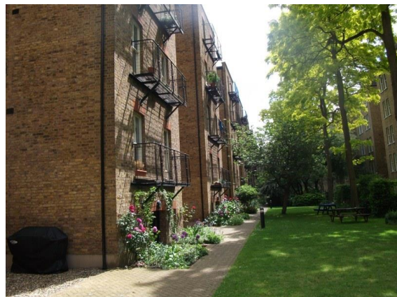
Balconies to rear of property.
