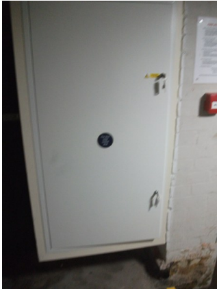
Appropriate signage on fire doors.
