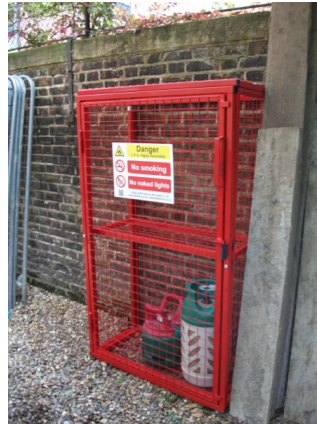
Designated cylinder cabinet outside block 1.
