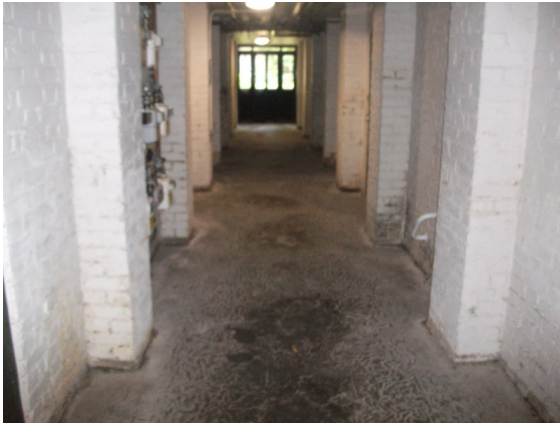
Example of basement corridor.
