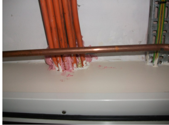
Example of fire separation in basement corridor services cupboard.
