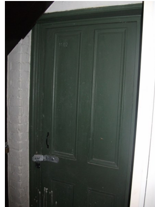
Example of locked door for residents' storage in basement area.
