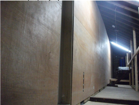
Roof space under development in block 10.
