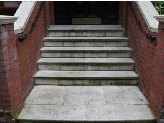
Example of block entrance steps.
