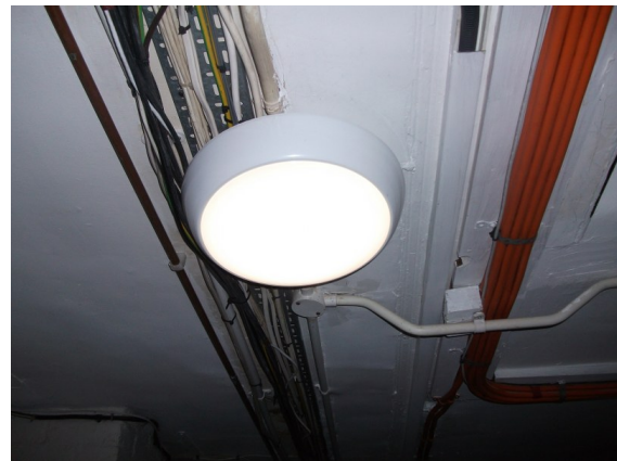
Example of artificial lighting in basement corridors.
